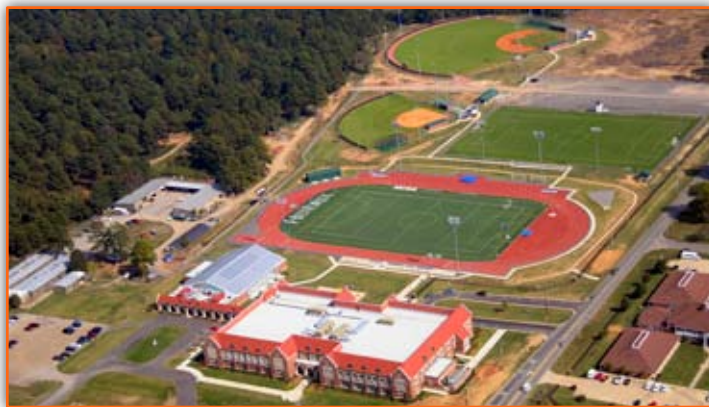
(Aerial view of the top-ranked Warrior facilities)
